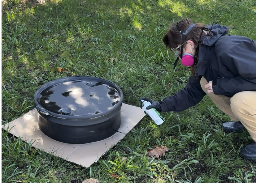
Figure 9.7: Lid section of the barrel being spray-coated with high-temperature rust-resistant paint; ports are taped off to protect against accidental sealant coverage.
