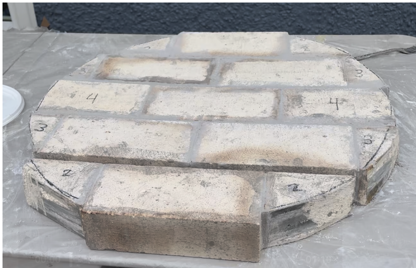
Figure 9.5: End slab masonry in progress, showing IFB pieces assembled to form the kiln lid and bottom hot faces.
